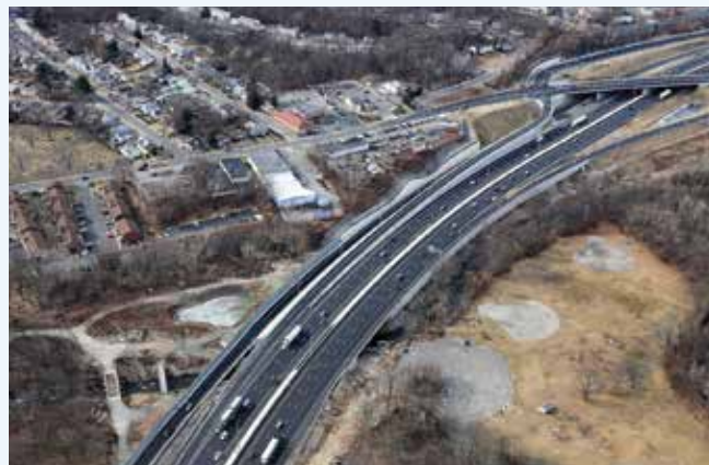
Adding a lane on I-84 provided for lane continuity.
