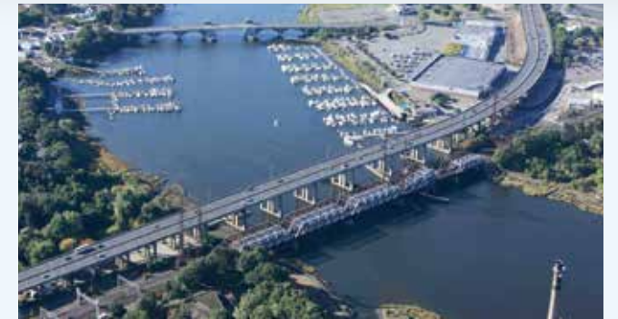
Reconstruction of the Moses Wheeler Bridge.
