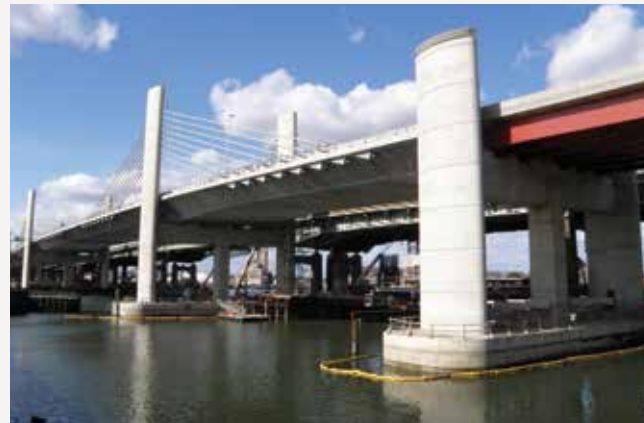
Reconstruction and widening of the Q Bridge.
